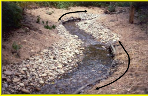
Completed LUNKERS after Construction
