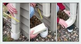
Disconnecting your downspout is a simple and effective way of reducing stormwater runoff. (Photo from grandbuilding.ca)
