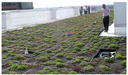
Figure 5. Modular Green Roof System Installation
