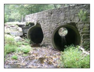
SC-01 is a twin 72-inch culvert for the stream crossing at Strobel Road, marking the beginning of the reach.
