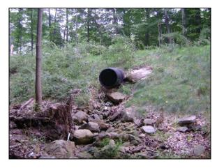
Tributary outfall OT-01 has an approximately 3-foot drop to the channel which is causing erosion and scour around the outfall.
