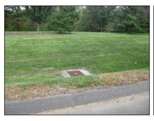
The catch basin is located in a grass swale to allow for infiltration prior to entering the storm drainage system.
