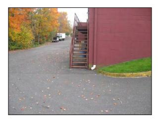
Downspouts discharge to impervious surfaces at Chuck's Corner Shopping Center.
