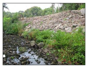
ISL-03B is channelized with rip-rap and placed stone in the stream channel.
