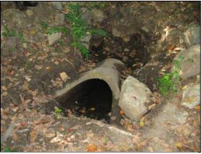
The concrete flared end segment of outfall OT-04 has collapsed and is no longer connected to the storm system.
