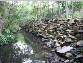
The biggest problem along reach ISL-04 is impacted buffers on residential properties. Many structures are built close to the stream bank (left) and a stone wall was constructed as a retaining wall to the river (river). Buffer encroachment prevents adequate connection to the floodplain.
