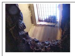
Storm drains discharge directly to the culvert for Basset Brook.
