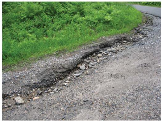
Eroded Shoulders - Install shoulder armor or create grassed swales.
