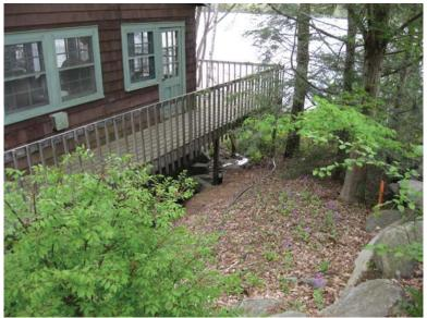
Drainage goes under existing deck & is flooding yard Insufficient room to create stabilized channel, Will require piping
