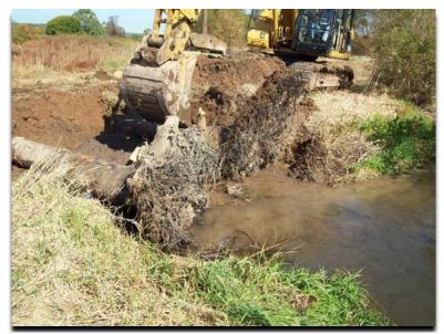
Figure 5.17: Rootwad Placement. Source: Princeton Hydro
