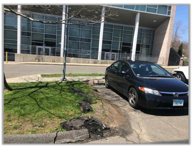
Figure 5.43: Another catch basin showing capture of leaf litter and solids from eroding lawn surface and poor state of repair for curbing
