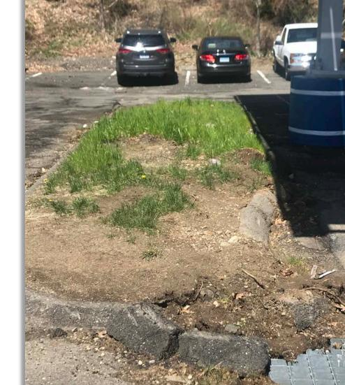
Figure 5.42: Parking lot catch basin inundated with eroding soils
