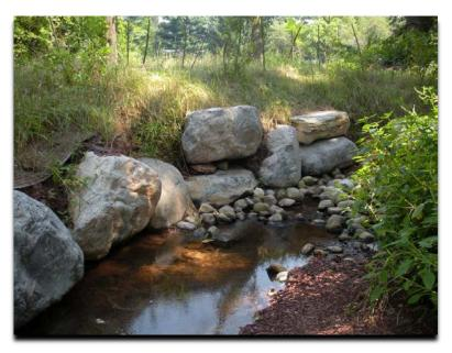
Figure 5.18: Boulder Toe Protection. Source: Princeton Hydro
