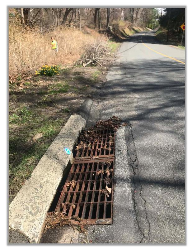
Figure 5.47: Beer Road catch basin to be retrofitted with basin insert
