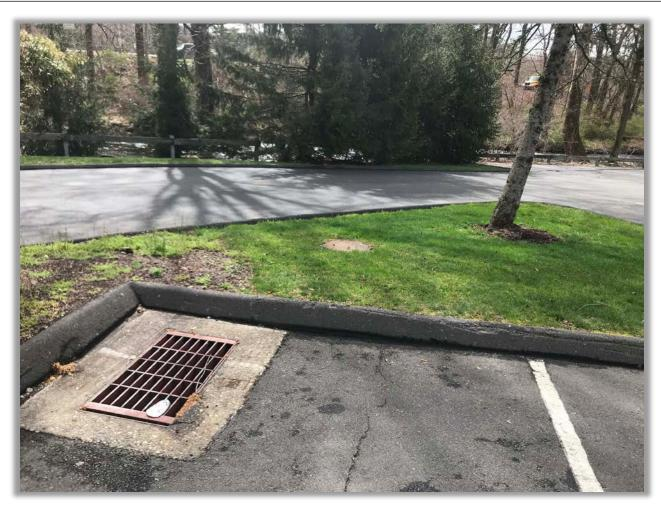
Figure 5.29: Target area for tree well unit; existing catch basin offers no stormwater treatment
