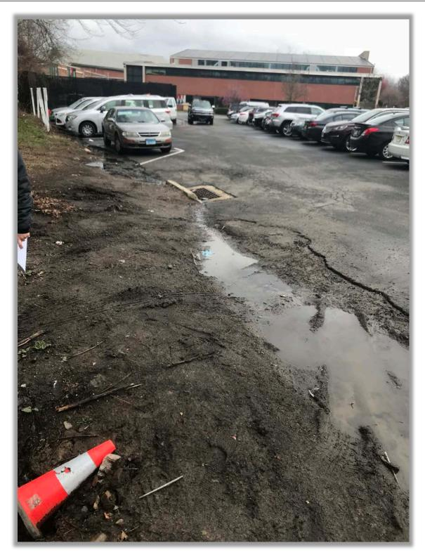
Figure 5.38: Poor stormwater management leads to ponding and generation of solids
