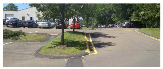
Figure 16. Tiered parking, with existing conveyances that transport stormwater from the upper tiers to lower tiers.
