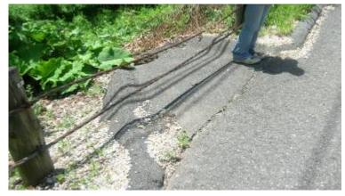
Curb Cut in Route 128 to Divert Stormwater Runoff Away from Travel Lanes
