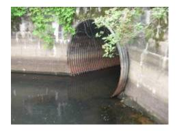
the headwall and the road grade together. However, the tree in the right hand photo above has an exposed root system which will kill the tree causing further bank erosion. The two photos below are of an outfall where one of two tributaries to Mill Brook crosses underneath Scoville Road. (This problem is occurring on the eastern most tributary). Because severe stream bank erosion is a problem here, it will be detailed in the Stream Bank Erosion Section below.
