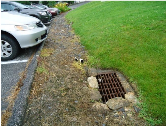
Photo 124: Parking Lot east of Old Building
