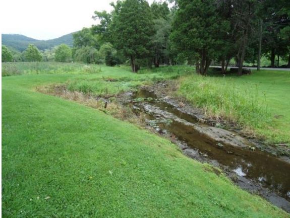
Photo 155: Inlet to School Pond (Lew's Lagoon)
