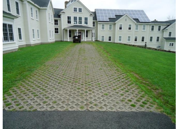
Photo 143: Grass pavers on a parking area in front of Gilder Hall Dormitory
