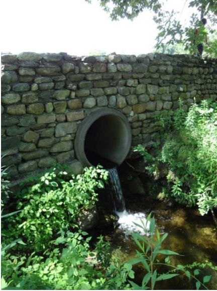
Photo 20: Stream Crossing at SKS entrance driveway
