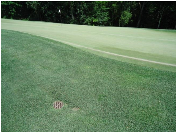
Photo 261 : Yard drain at Hole #5 that drains to a wetland on the opposite side of the green
