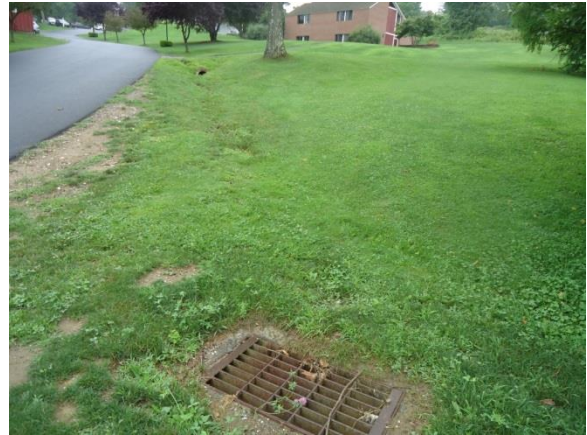
Photo 128: Drainage along roadway to Admissions Building
