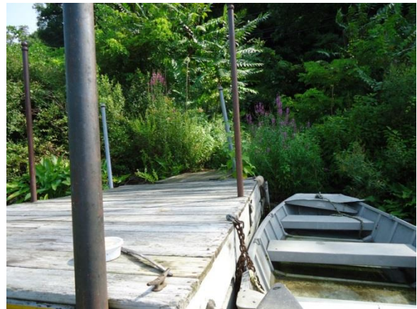
Photo 317: Dock along segment HP-06/07
