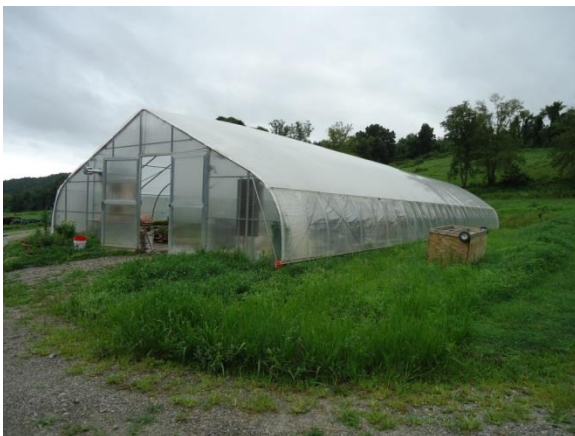
Photo 185: Greenhouse is used for plants and equipment storage, which limits the amount of outdoor storage and minimizes contact with stormwater
