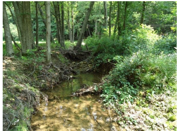
Photo 106: Bank erosion evident along segment SM-01A
