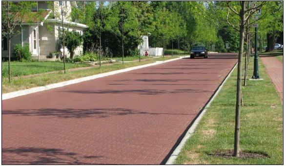
*Figure 8-12. A residential pervious paver road (Image from Pine Hall Brick Company, Inc.* <u>www.pinehallbrick.com</u>).
