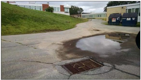
*Figure 8-41. Deposition of eroded sediment near a catch basin at the school delivery area.*
