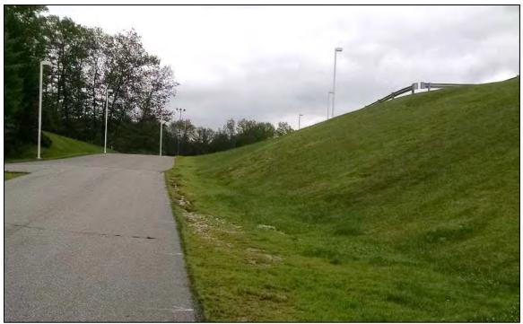
Figure 8-32. Erosion at the toe of the slope along the driveway to the high school.
