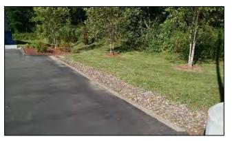
A gravel strip at the edge of the parking area at Dollar General filters stormwater before it enters a grassed swale that leads to an infiltration basin at the rear of the property.
