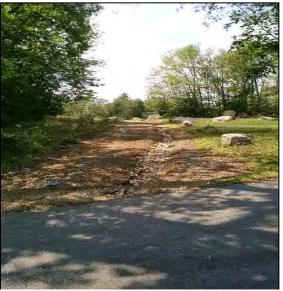
Uncontrolled stormwater runoff from a commercial property in North Grosvenordale has resulted in the development of a deep gulley and deposition of the eroded sediment in the street down-gradient of this dirt driveway.
