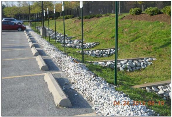
Figure 8-35. Example of check dams placed in a grass swale to slow water flow and prevent soil erosion (image - <u>www.chesapeakestormwater.net</u>).
