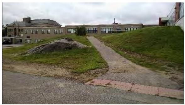
*Figure 8-39. Erosion along a walkway and sediment deposition near the school delivery area.*
