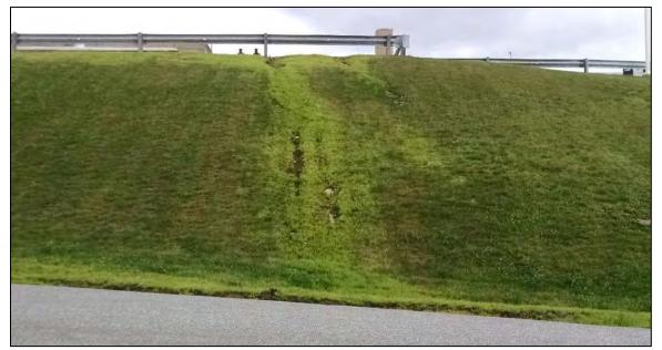
*Figure 8-33. Erosion on the hillside along the driveway to the high school caused by stormwater runoff from the parking lot at the top of the slope.*
