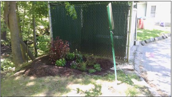
Figure 8-1. A rain garden installed at Moosup Garden Apartments to infiltrate contaminated runoff from the adjacent dumpster.
