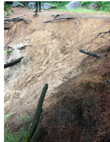
Photo 2-3: Sandy soils eroding into Bantam River.
