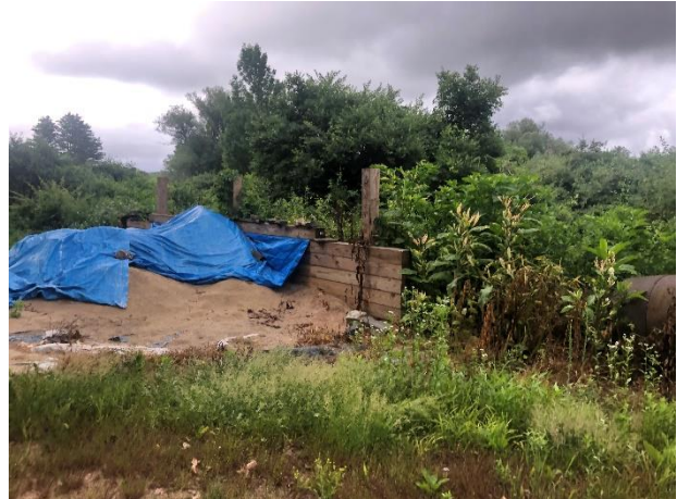
Photo 4-7: Soil stockpile partially covered with a tarp.
