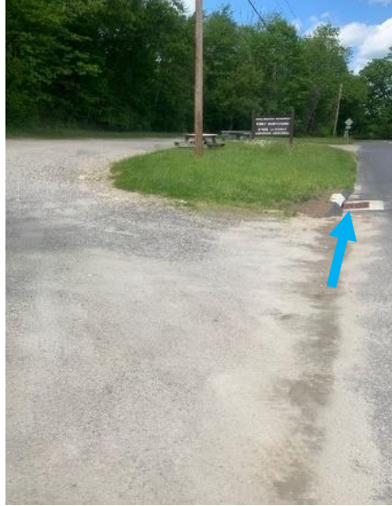
Photo 8-2: Campground store parking lot with catch basin.
