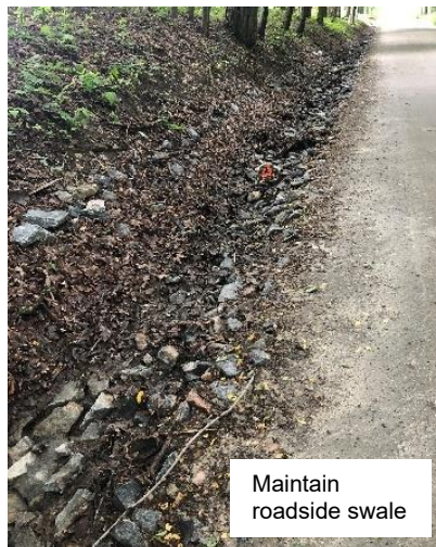
Photo 6-2: Roadside swale installed by Goshen DPW.
