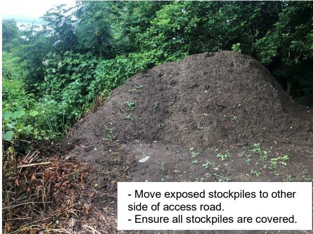
Photo 4-6: Exposed soil stockpile at LCC3.
