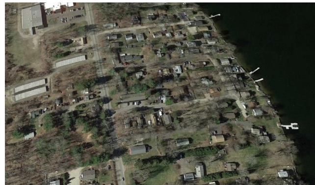
Photo N2-1: Neighborhood off of Route 209
