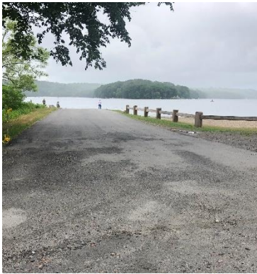
Photo 7-1: Road leading down to boat launch.
