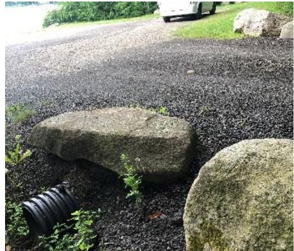
Photo 5-2: Culvert under gravel road at parking lot entrance.
