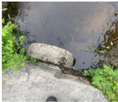
Photo 1-2: Downstream side of culvert discharges to Bantam River.
