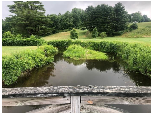
Photo 4-3: Upstream side of bridge at LCC1.
