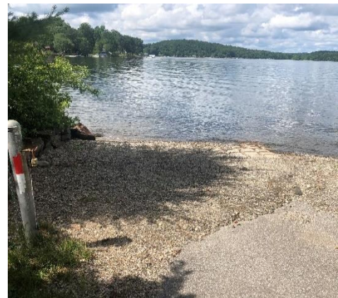
Photo 10-2 and 10-3: Erosion at boat launch to Bantam Lake.
