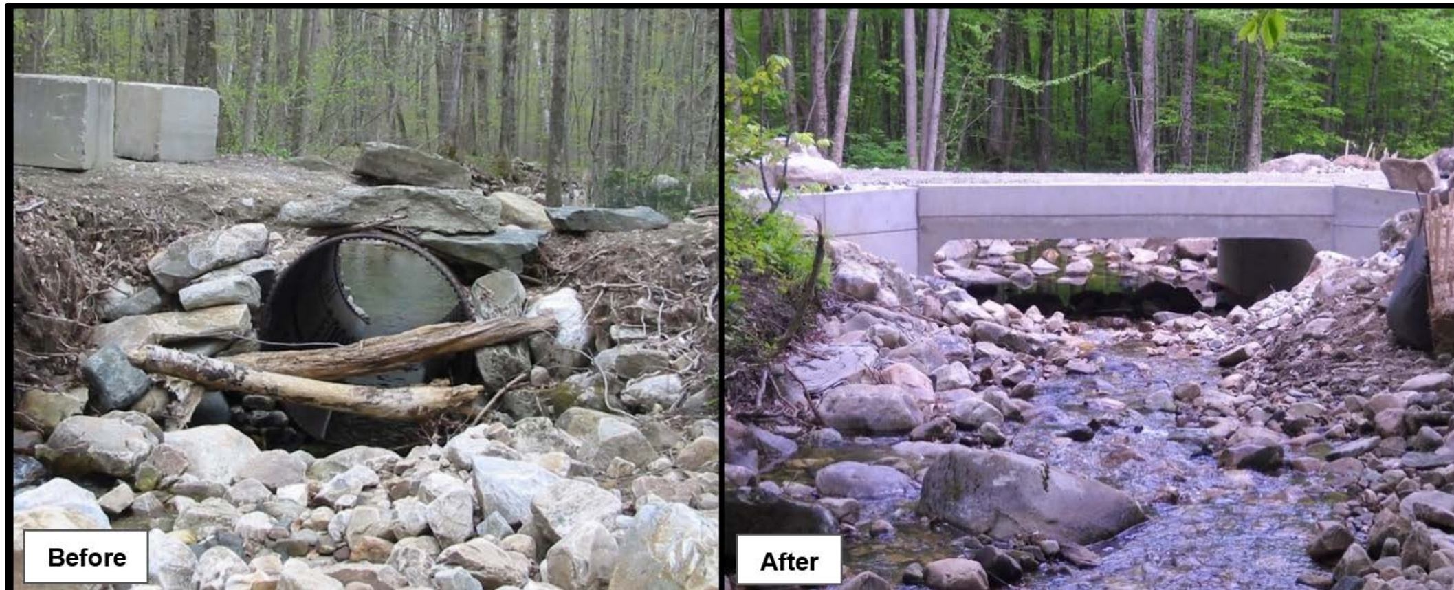
Example Culvert Replacement
