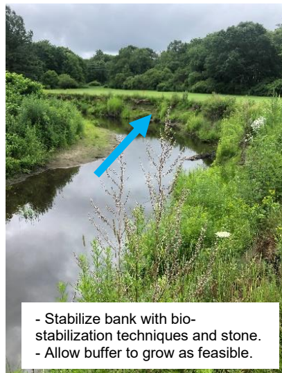
Photo 4-12: Eroding bank along Bantam River at LCC6.
