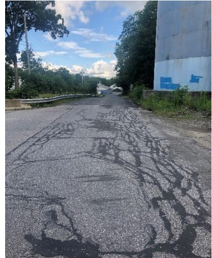
Photo C2-3: End of Russel Street at the entrance to the DPW yard.
