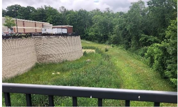
Photo C1-2: Stop-n-Shop Plaza, adjacent to parking lot
