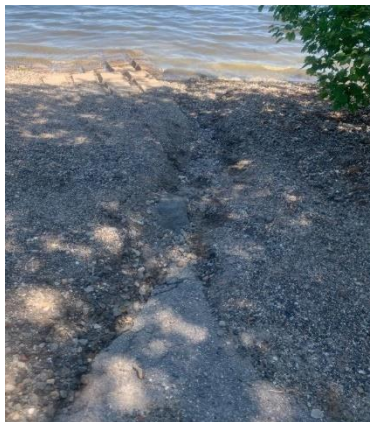
Photo 10-2 and 10-3: Erosion at boat launch to Bantam Lake.
