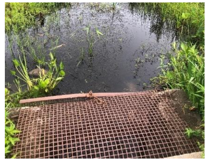
Photo 1-3: Top of upstream side of culvert draining wetland.
