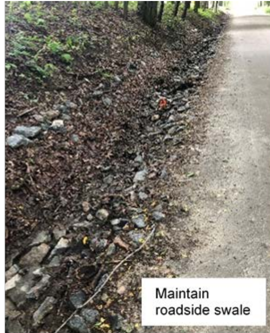
Photo 6-2: Roadside swale installed by Goshen DPW.
