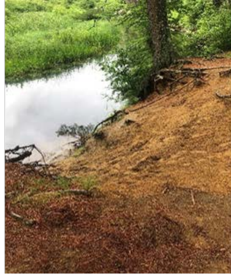
Photo 2-2: Severe erosion at site.
