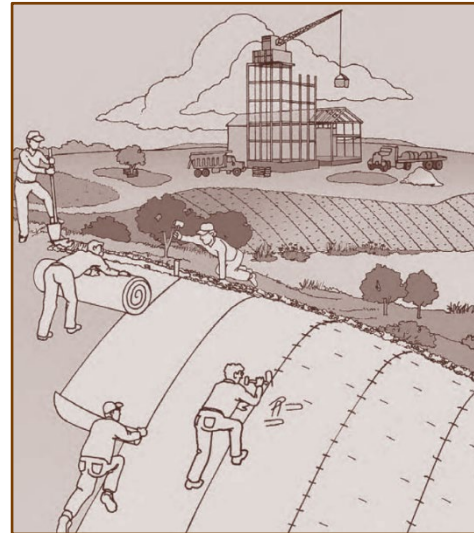
Figure 5- 13 Example of Temporary Erosion Control Blanket Installation
