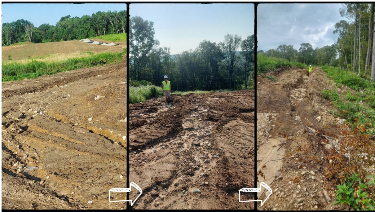
Figure 2- 2. Gully Erosion and the Possible Progression
