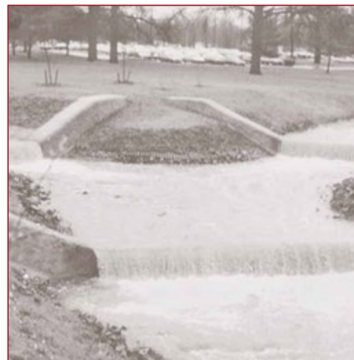
Figure 5- 24 Example of a Grade Stabilization Structure
