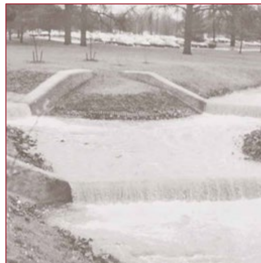
Figure 5- 24 Example of a Grade Stabilization Structure
