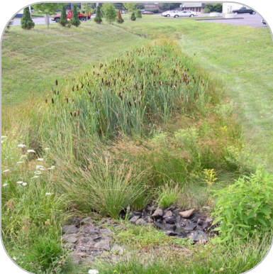
Water Quality Conveyance BMPs
