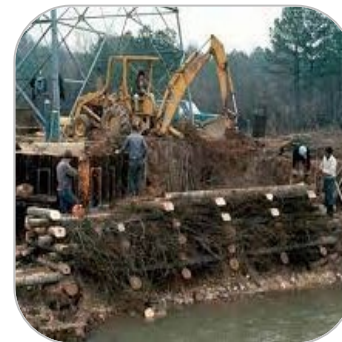
Live Crib Walls
