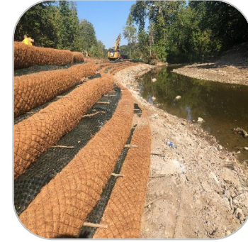
Bioengineering Fiber Rolls
