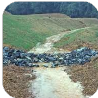
Stone Check Dam
