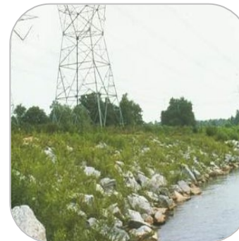
Joint Planted Revetment
