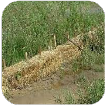
Hay Bale Barrier (Replaced with Straw Bales)
