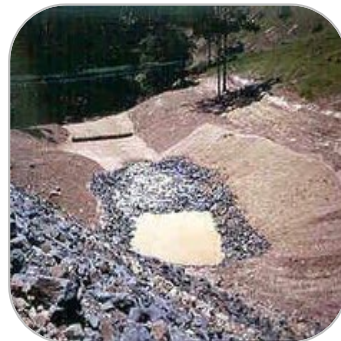
Temporary Sediment Basin
