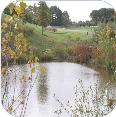
Stormwater Pond BMPs
