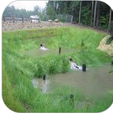
Stormwater Wetland BMPs
