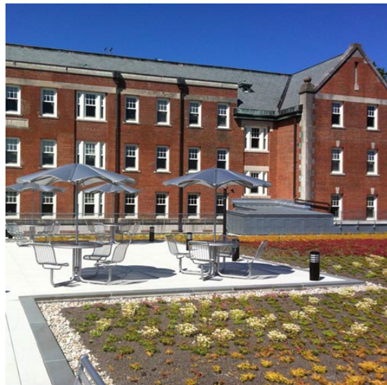
Simple Intensive Green Roof, Storrs Hall, Storrs, CT
