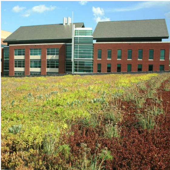
Extensive Green Roof, Laurel Hall, Storrs, CT
