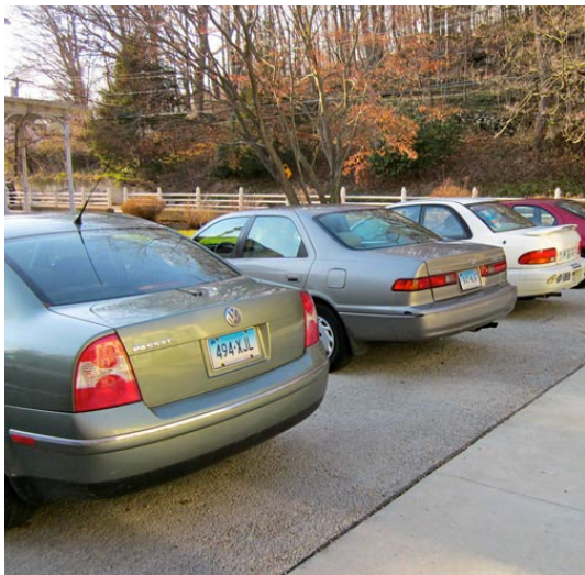
Pervious Concrete (Residential Subdivision, East Haddam, CT)
