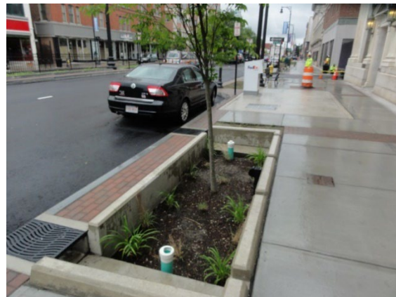
Bioretention planter in urban downtown setting.
