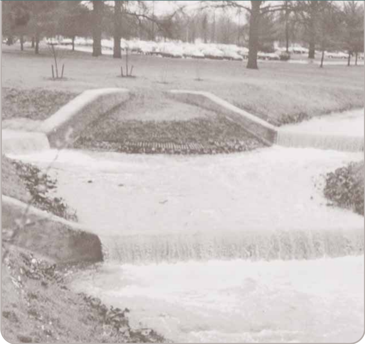
Figure CSS-I Example of Grade Stabilization Structure
