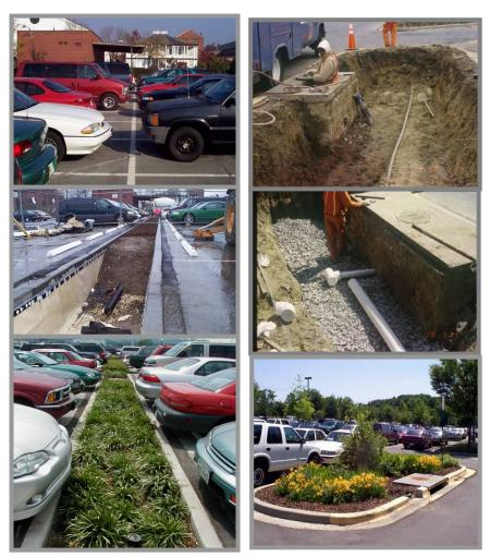
Figure 4.15 – Bioretention retrofit at the U.S. Navy Yard in Washington, D.C.
