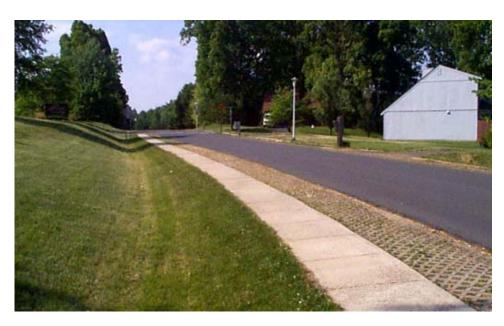
Figure 4.7 - Narrow road section with sidewalks, shallow swale and porous pavement shoulders.
