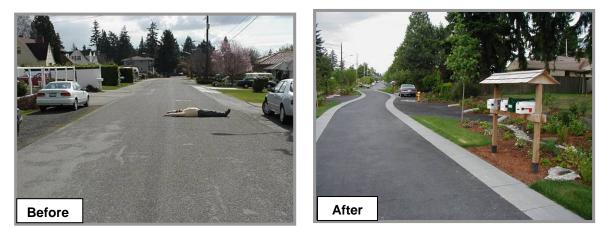
Figure 4.17 – LID urban retrofit project in Seattle, WA, using rain gardens/detention cells.
