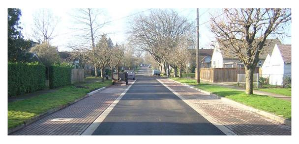
Figure 4.13 – Porous surfaces.
