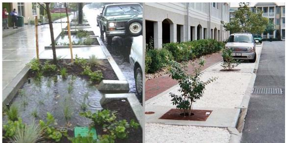
Figure 4.12 – Examples of planter box designs in high density development.
