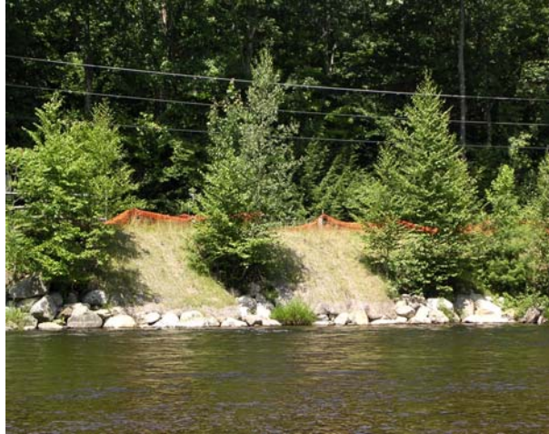
After Stabilization Project
