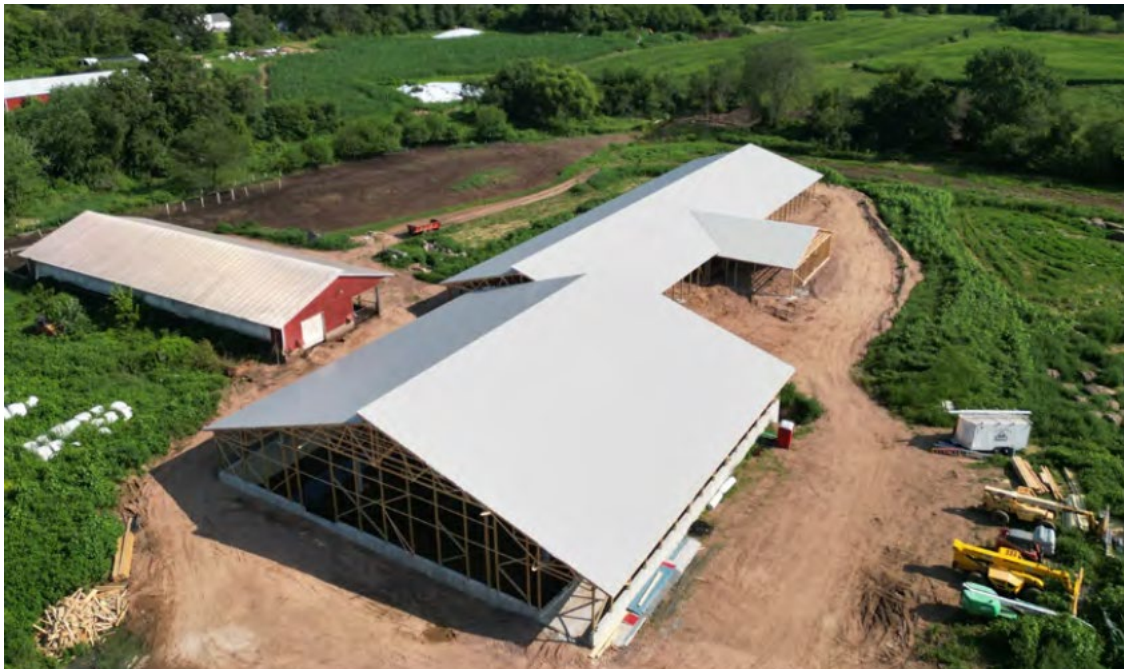
Figure 6 Drone footage of the newly constructed free-stall barn and waste storage structure. Image courtesy of NCCD.
