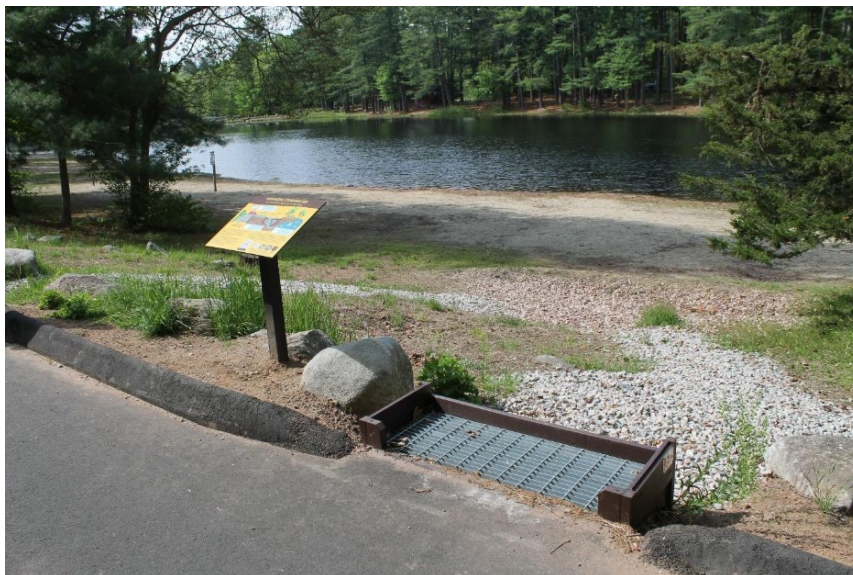
Figure 15: BMP and signage installed at Chatfield Hollow State Park.
