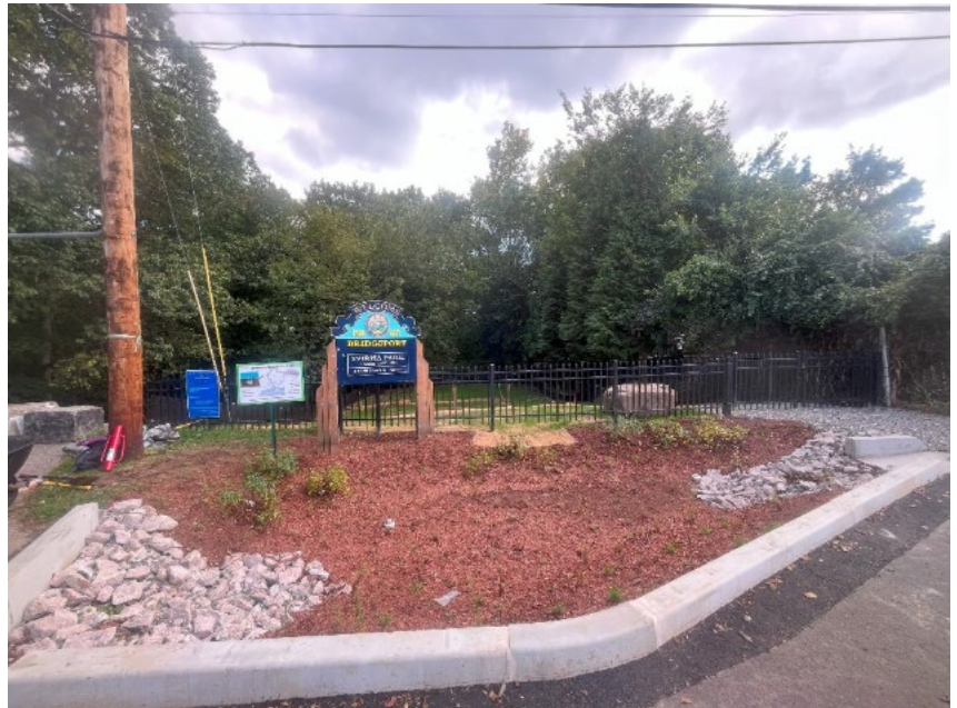
Figure 1 Bioretention system at the entrance to Svihra Park. Image courtesy of The Nature Conservancy.
