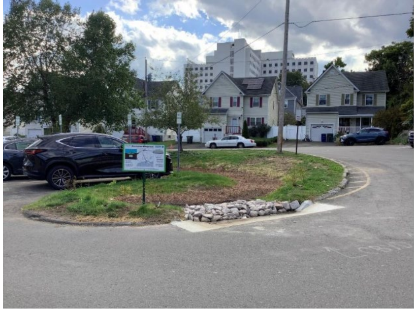
Figure 2 Bioretention system at Read School with curb inlet to divert stormwater from the adjacent parking lot and stone apron to dissipate energy as stormwater enters the area. Image courtesy of The Nature Conservancy.
