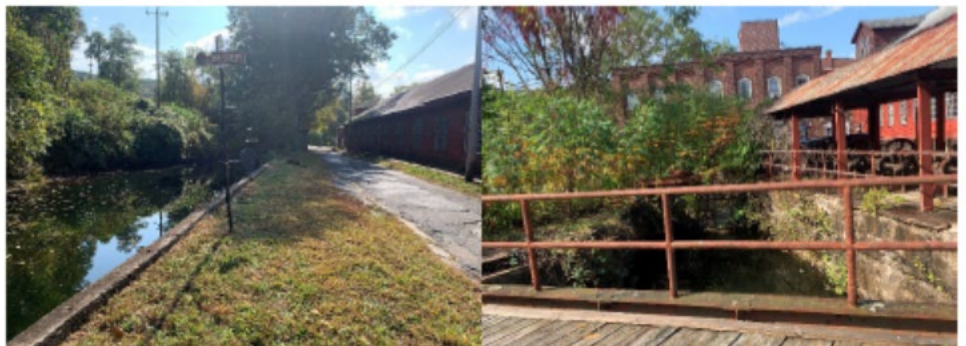
Figure 13 Images of the Collinsville Axe Factory in Canton from a site visit to determine whether the factory should be removed, set directly adjacent to a tributary to the Farmington River. Image courtesy of NCCD.
