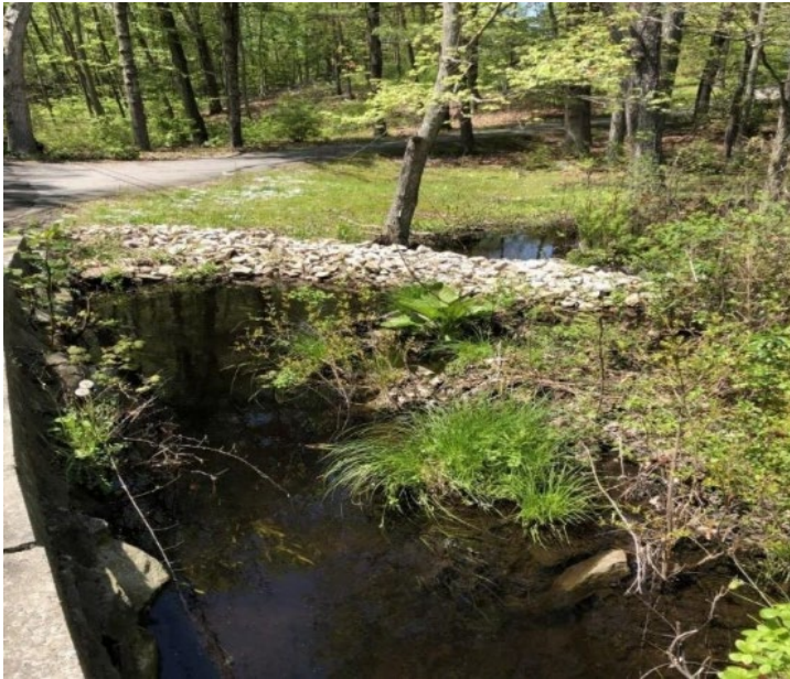
Figure 4: Impermeable berm installed across the bypass channel, directing flow into Christopher Pond. Image courtesy of The Town of East Hampton
