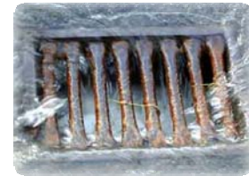
Stormwater drain near Quinnipiac River
