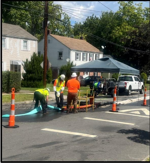
Lining project in North Hartford to help reduce flooding issues in the area
