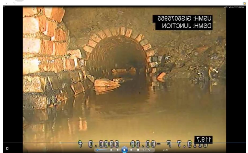
Sewer collapse in a combined sewer in Hartford resulting in a discharge
