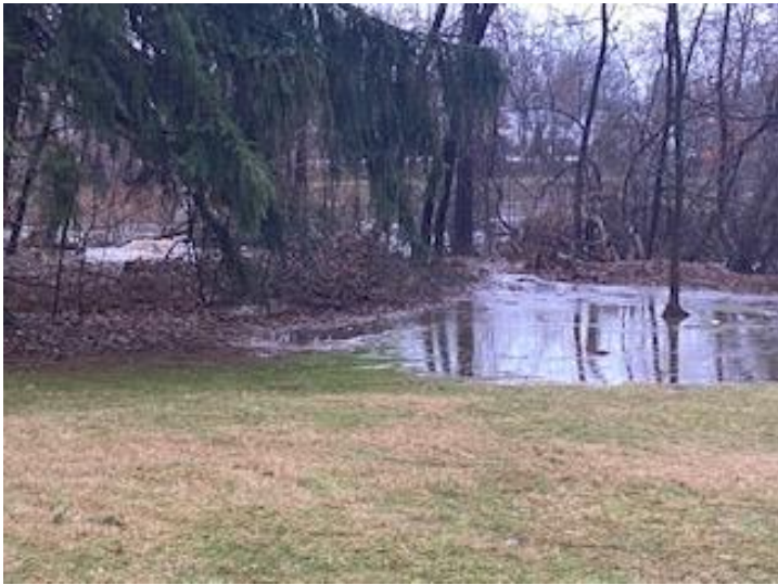
Sewage overflow from a manhole in a backyard
