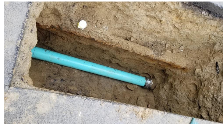
Deformed/broken pipe replaced with PVC pipe and shielded banded couplings
