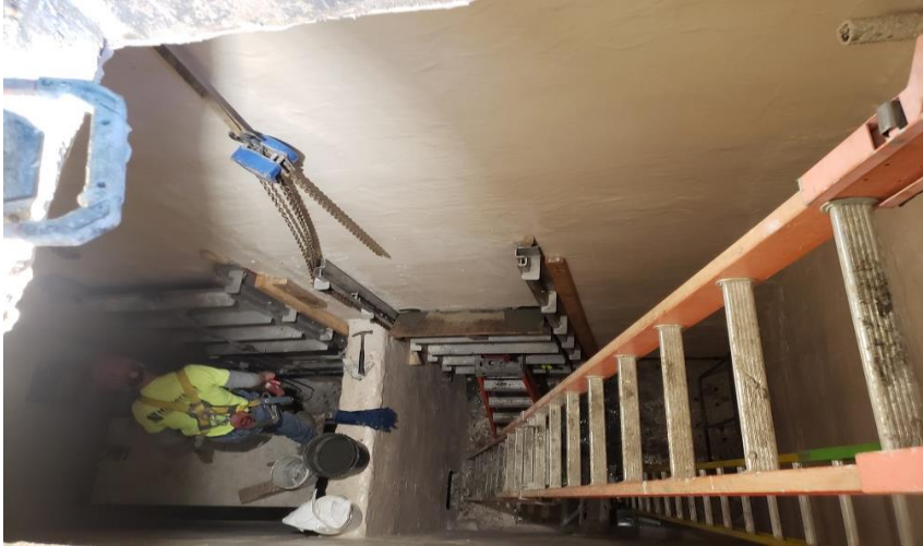
Fort Point PS Wet Well Coating
