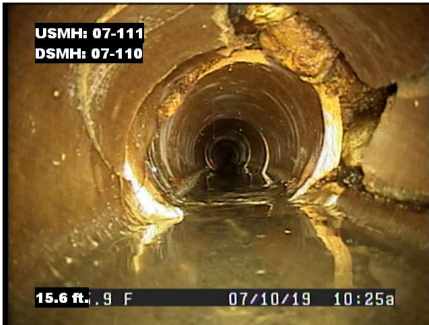
Pre Lining – 8-inch VCP Midrocks Drive – Easement
