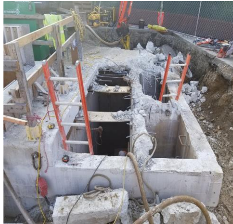
Wet Well Concrete Work
