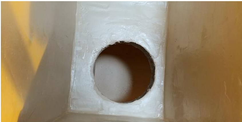
Westport Ave PS Wet Well Coating
