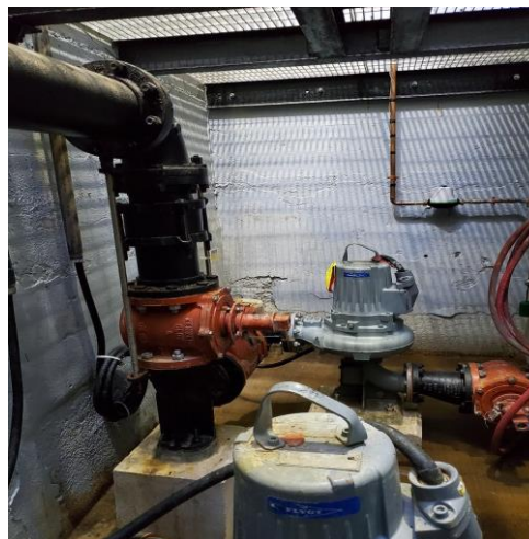
New Flygt Dry Pit Pumps and Piping
