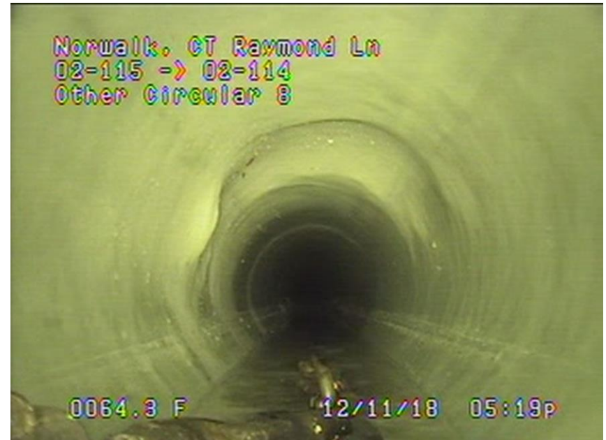
Post Lining Raymond Street
