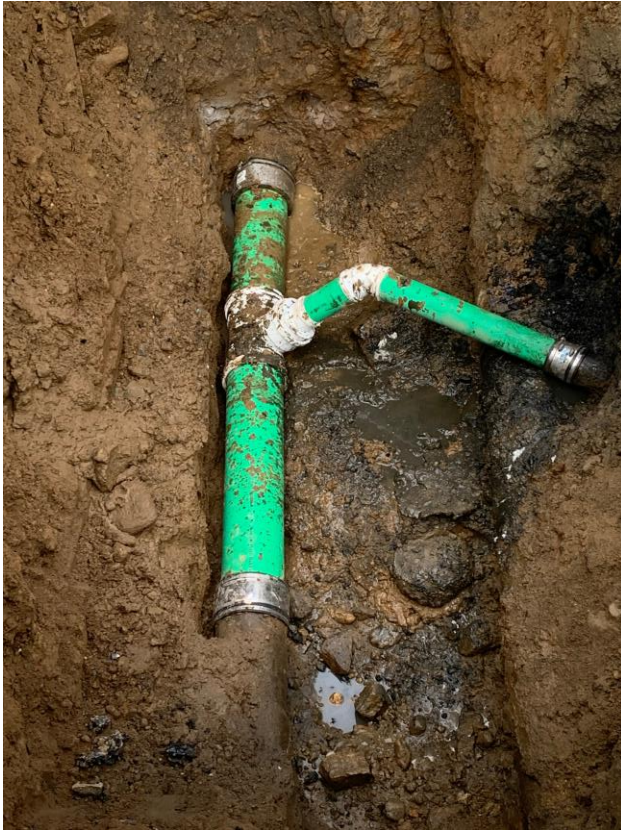
Deformed/broken pipe replaced with PVC pipe and shielded banded couplings
