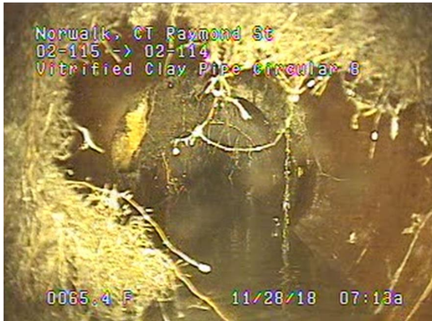
Pre Lining – 8-inch VCP Raymond Street
