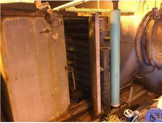
94. Pipe Gallery former air handling unit with suspect HBM..
