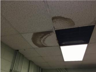
21. Screen Building control room with stained/damaged ceiling tiles/suspect HBM.
