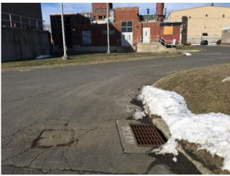
116. Typical Site catch basin connected to sanitary sewer system.
