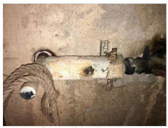
89. Pipe Gallery pipe insulation and suspect ACM.
