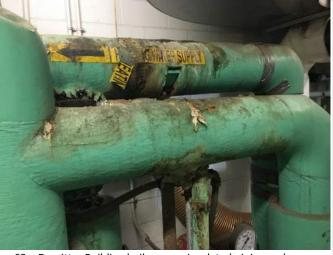
68. Degritter Building boiler room insulated piping and suspect HBM.
