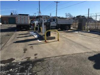
112. The Site's fuel station with one 5,000-gallon gasoline and one 5,000-gallon diesel UST.
