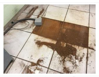
22. Screen Building control room with stained/damaged floor tiles/suspect HBM.
