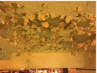
90. Pipe Gallery peeling paint and suspect lead paint.
