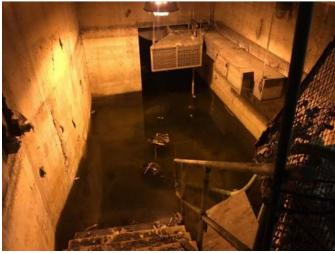
41. Pump Station basement, flooding, and suspect HBM.
