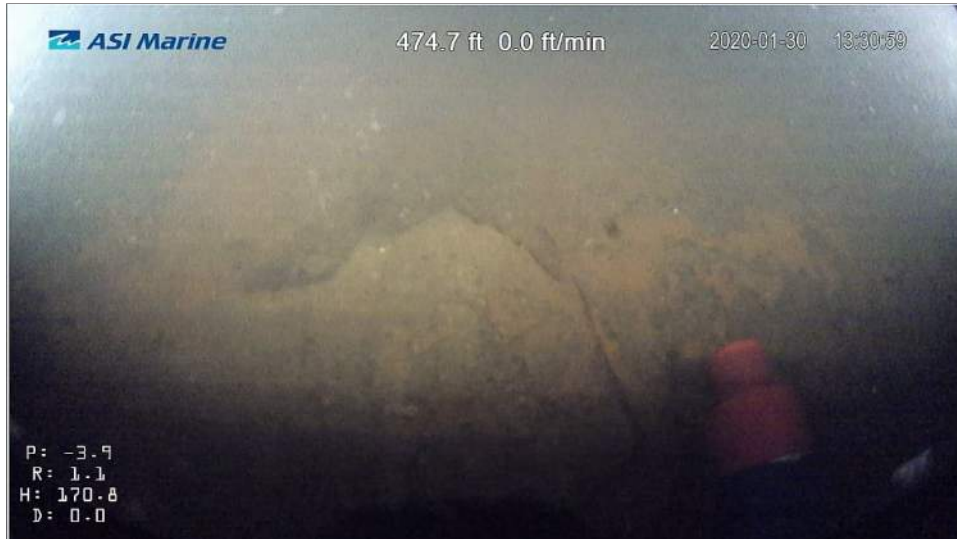
Image 4.2.1-19: Image of invert 475 feet downstream of Access Point 1.
