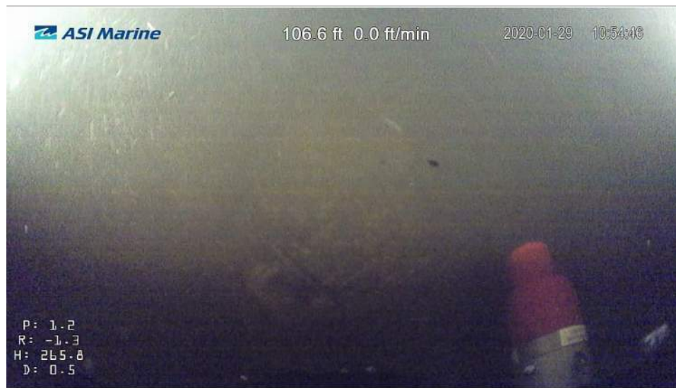
Image 4.1.1A-2: Feature on invert at 107 feet downstream of Manhole 1.
