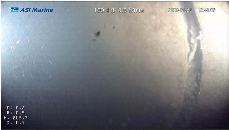
Image 4.1.1B-4: Image of joint 100 feet downstream of Manhole 3.
