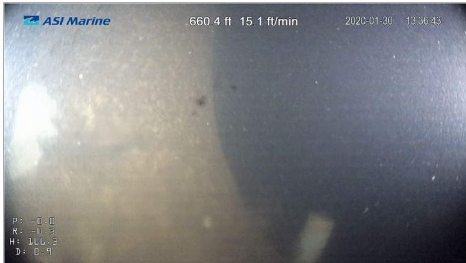
Image 4.2.1-24: Image of debris 660 feet downstream of Access Point 1.
