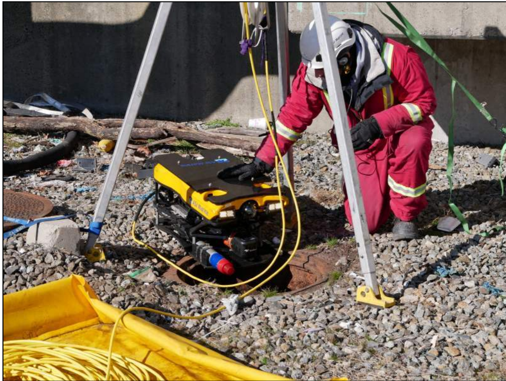
Figure 7: ROV at Manhole 3
