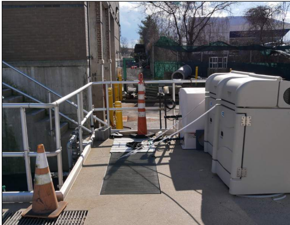
Figure 8: Access Point 1 at the West plant chlorine contact tanks
