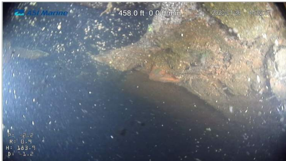
Image 4.2.1-18: Image of crown 458 feet downstream of Access Point 1.
