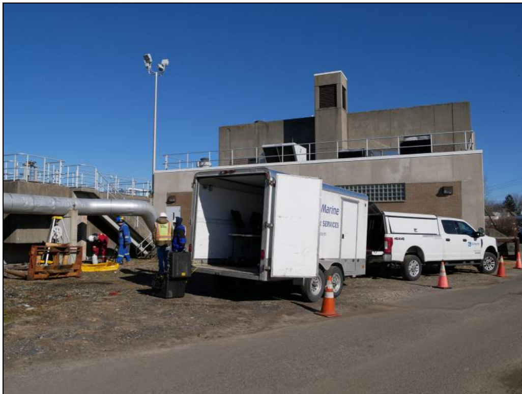
Figure 6: ASI truck and operations trailer adjacent to Manhole 3
