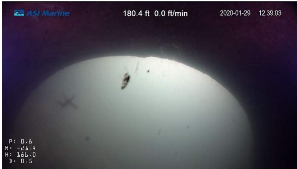
Image 4.1.1B-9: Outfall 180 feet downstream of Manhole 3.
