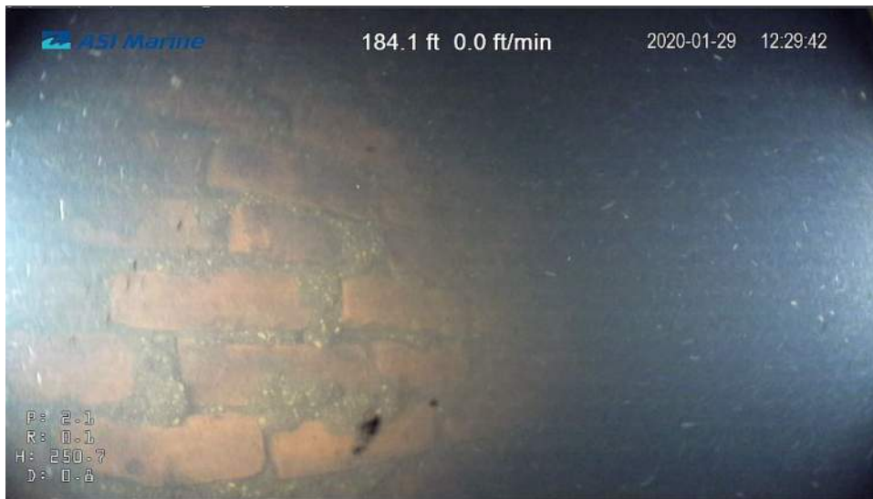
Image 4.1.1B.10: Outfall structure 184 feet downstream of Manhole 3.
