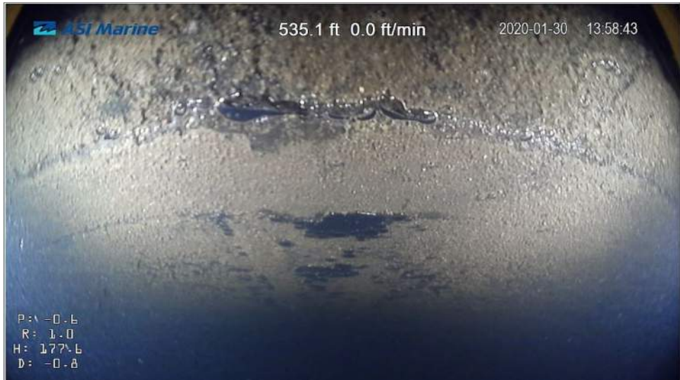
Image 4.2.1-21: Image of joint 535 feet downstream of Access Point 1.
