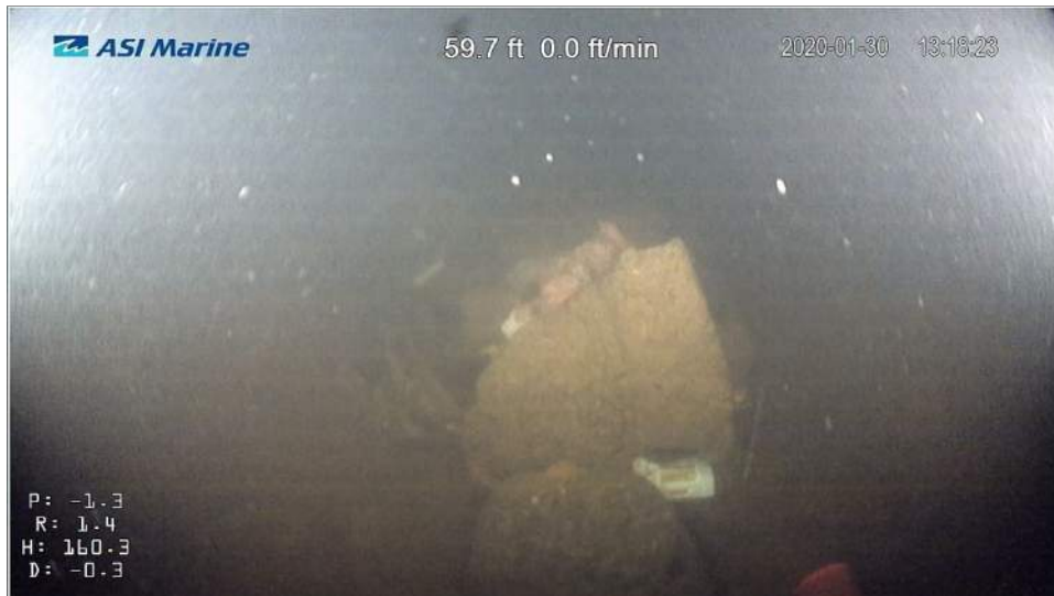
Image 4.2.1-2: Debris on invert 60 feet downstream of Access Point 1.
