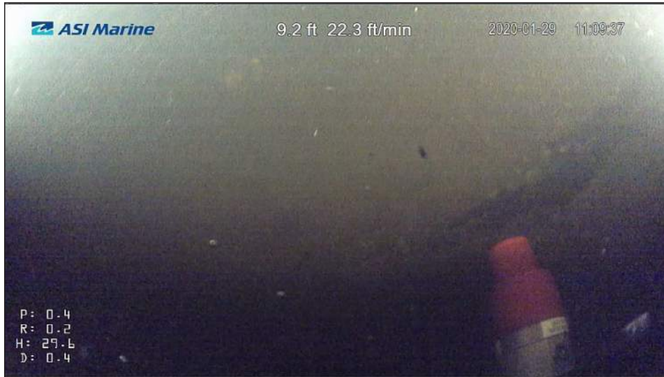
Image 4.1.1A-6: Image of joint at invert 9 feet upstream of Manhole 1.
