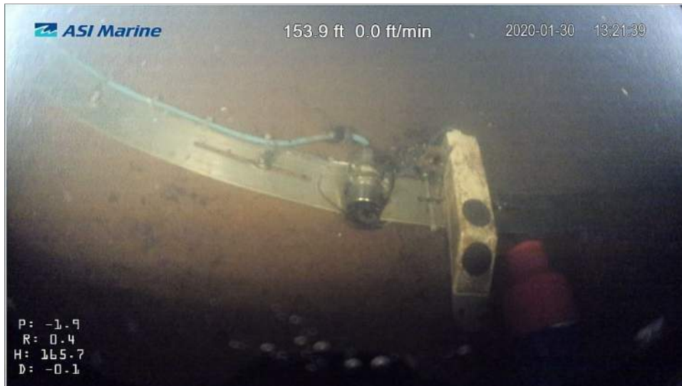
Image 4.2.1-8: Instrumentation on invert 154 feet downstream of Access Point 1.
