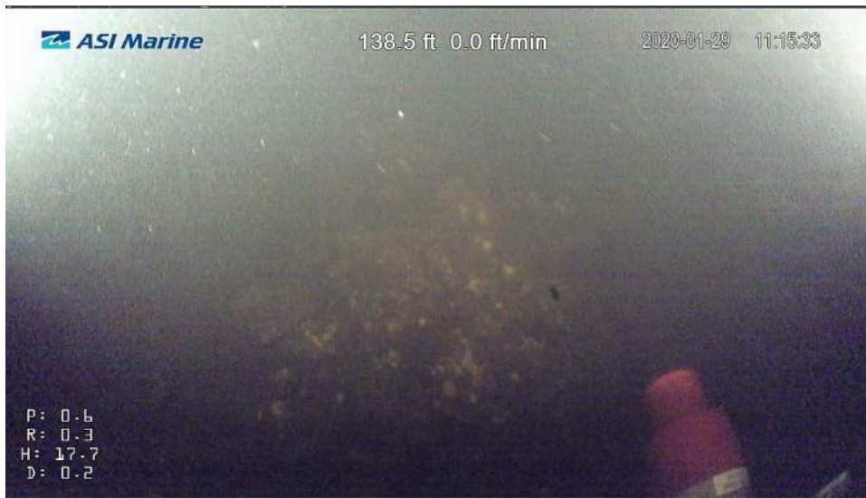
Image 4.1.1A-14: Debris on invert 138 feet upstream of Manhole 1.
