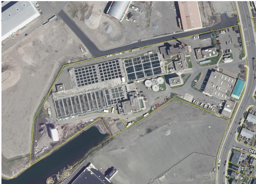
Figure ES-4 Aerial of East Side Wastewater Treatment Plant
