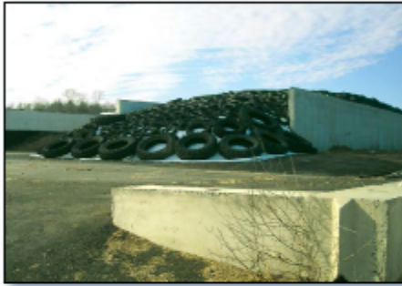
Figure 2. The completed silage bunker and leachate collection system helps to manage manure at Valleyside Farm in Woodstock, Connecticut.
