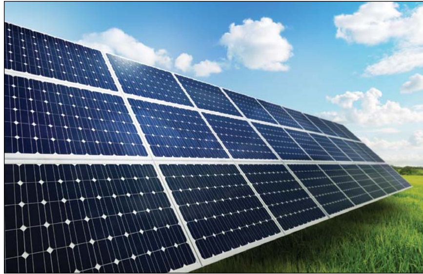
The closed Hartford landfill will soon feature one of Connecticut's largest solar-panel arrays, strengthening CRRA's goal of providing renewable power to the state's residents.
