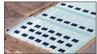
A flexible solar array uses special photovoltaic material built right into the cap. So the landfill itself would become a solar-power collector.
