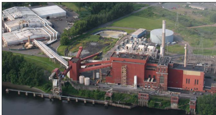
The Mid-Connecticut plant in Hartford is the center of our trash-to-energy system.
