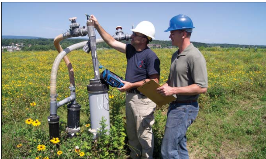
Continual monitoring of the gas collection system at closed landfills helps protect area residents and the environment from undue health hazards.
