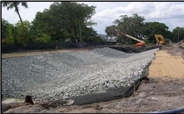
Recycled concrete for erosion control
