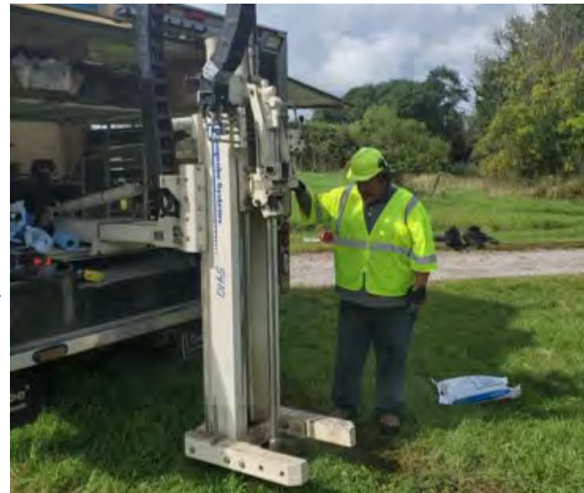
INSTALLATION OF BORINGS & WELLS
