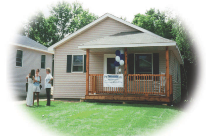
A new home built on a former brownfield in the Twin Cities area, Minnesota.
