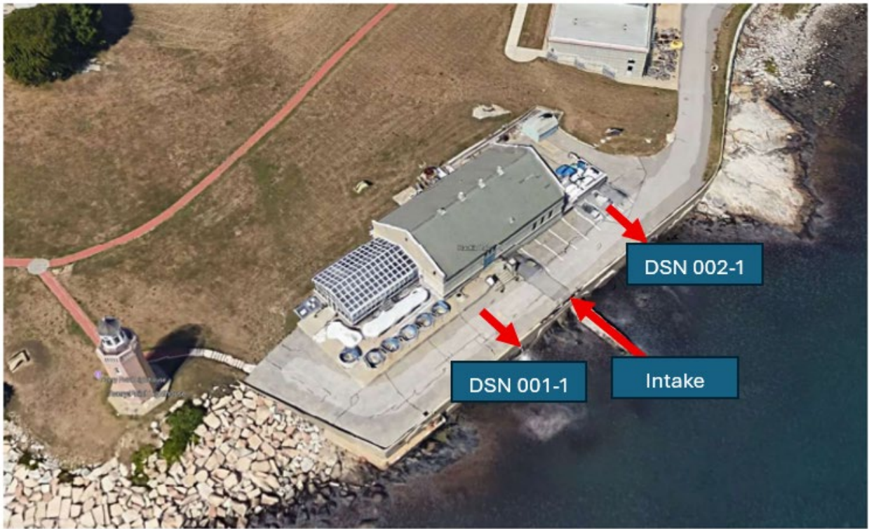
Figure 2.1. Image of discharge locations
