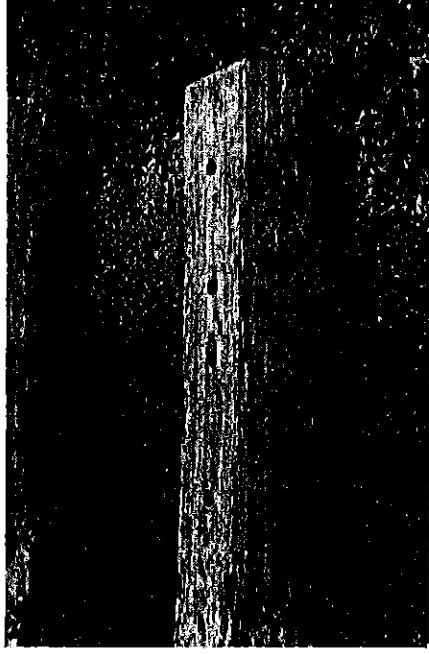
Figure 19 Boring prior to treatment.
