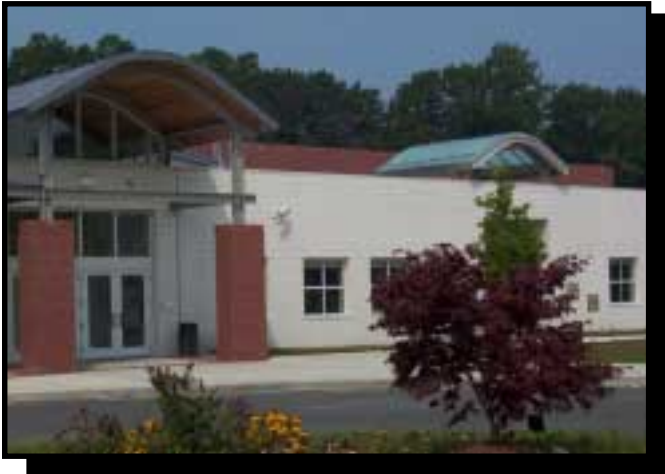
McKinley School in Fairfield benefits from daylighting
