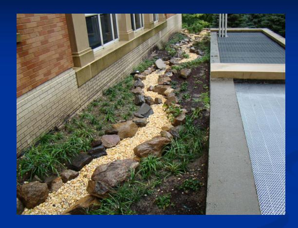
Mitigation of Stormwater runoff into grid area
