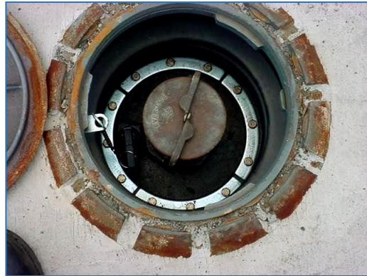
Example of a clean spill bucket.
