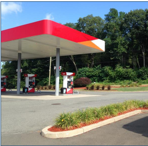
A canopy over the pumps prevents stormwater washing away contaminants. The fueling area is paved with nonporous concrete.
