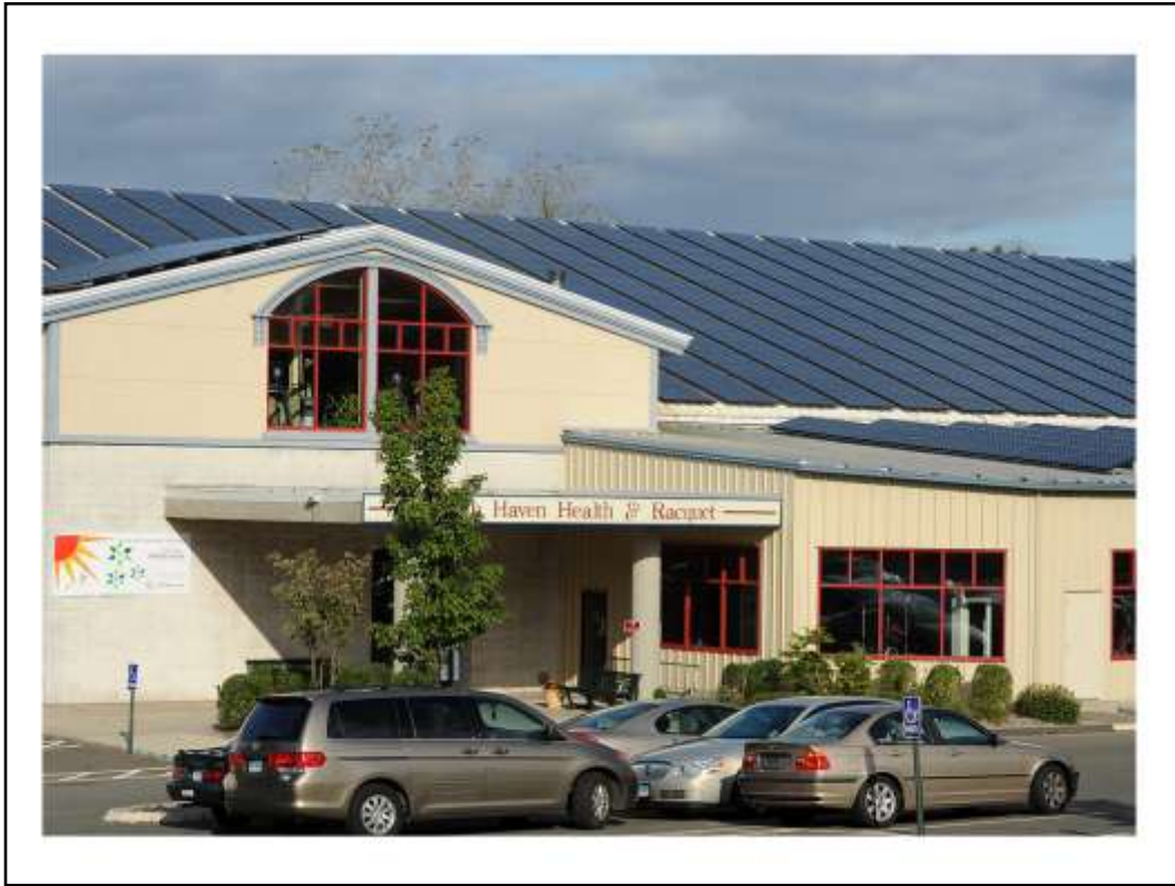
22 thousand S/F 826 panels 230 watts each were installed at one of the other family owned properties buildings
