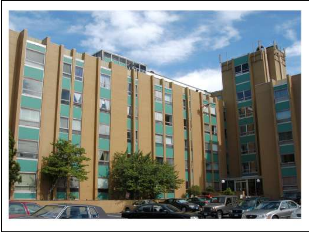
Lakewood, Apt. 130 units, New chiller reduced electrical by 44%, new boilers saved 15% FUEL SAVING, adding solar thermal
