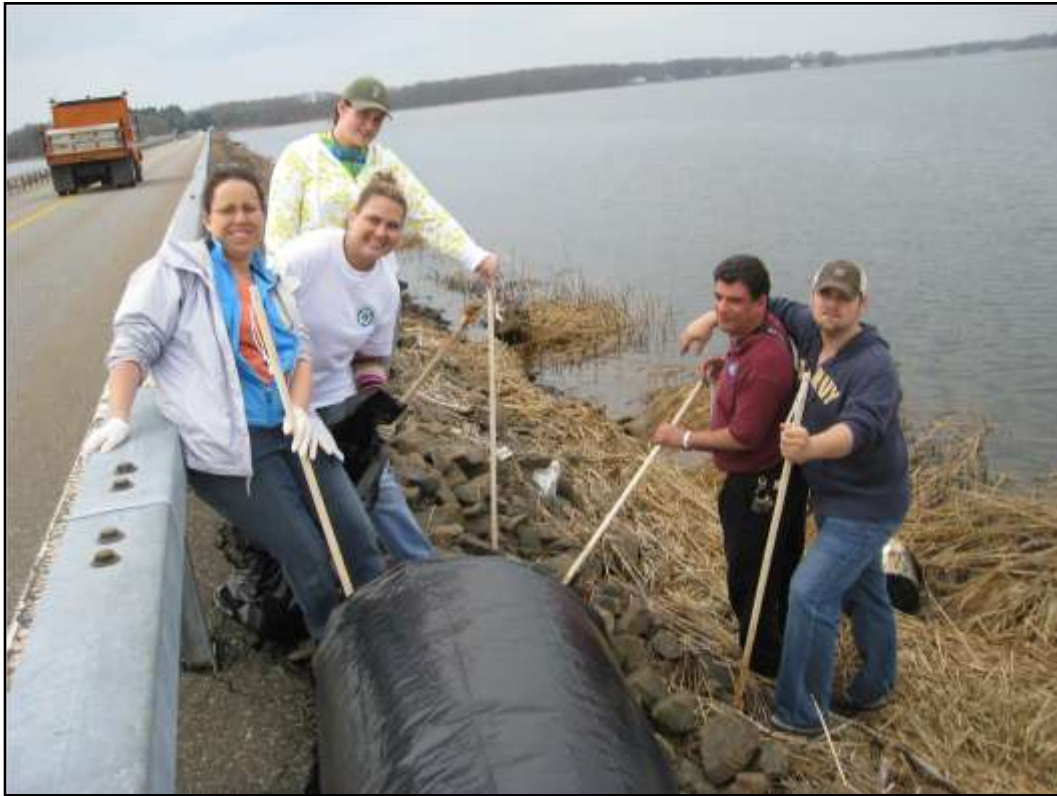
Bridge St, scenic highway Rt. 154 South Cove.
