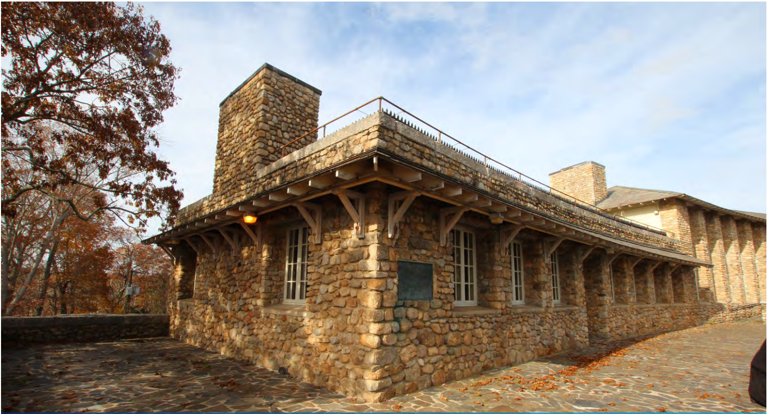
Terrace and rooftop terrace
