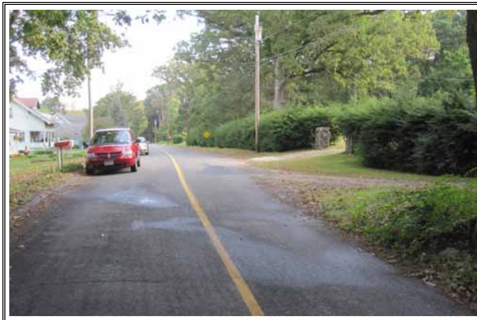
Northern view of subject's High Street frontage (on right)
