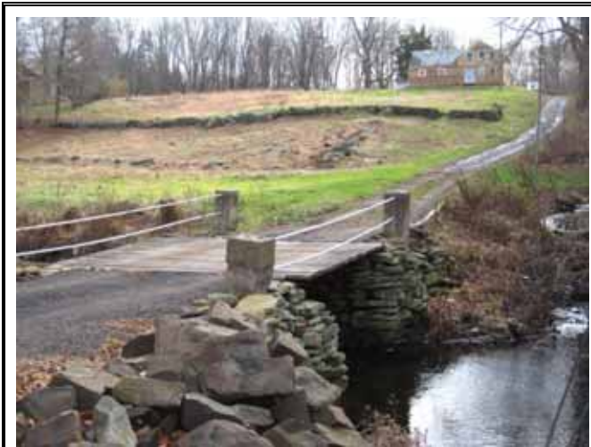
Access bridge from Old Marlborough Turnpike
