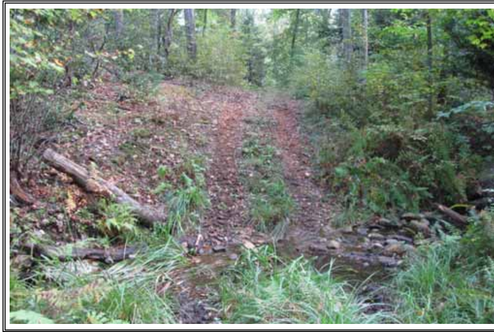
Interior view of stream crossing and logging road
