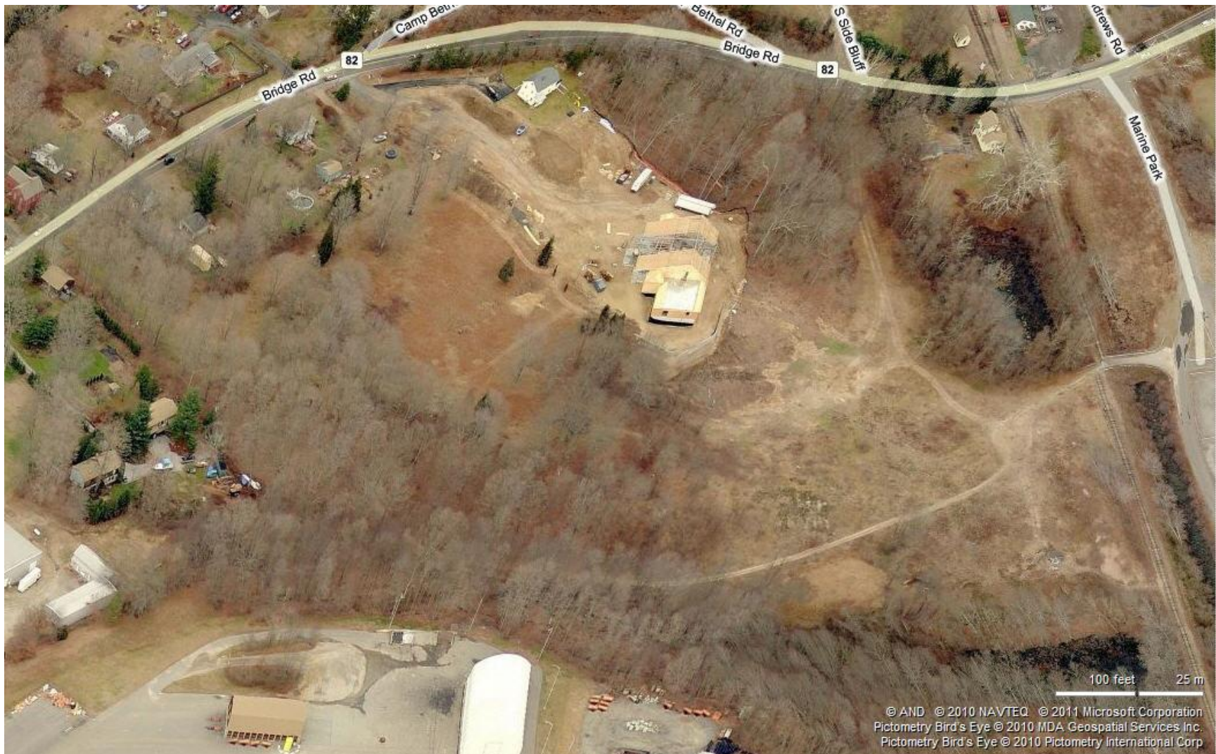
Undated oblique aerial photograph to the north showing the subject property and adjacent banquet facility under construction (Source: Bing Maps)
