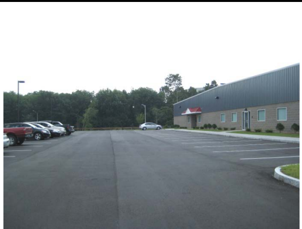
Southerly view of retail section towards I95
