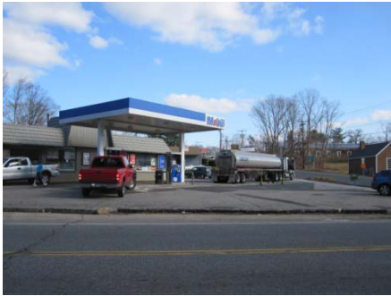
Easterly view of gas station/convenience store at corner of Rt. 82 and Rt. 154
