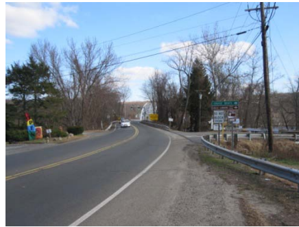
Easterly view of bridge from Rt. 82
