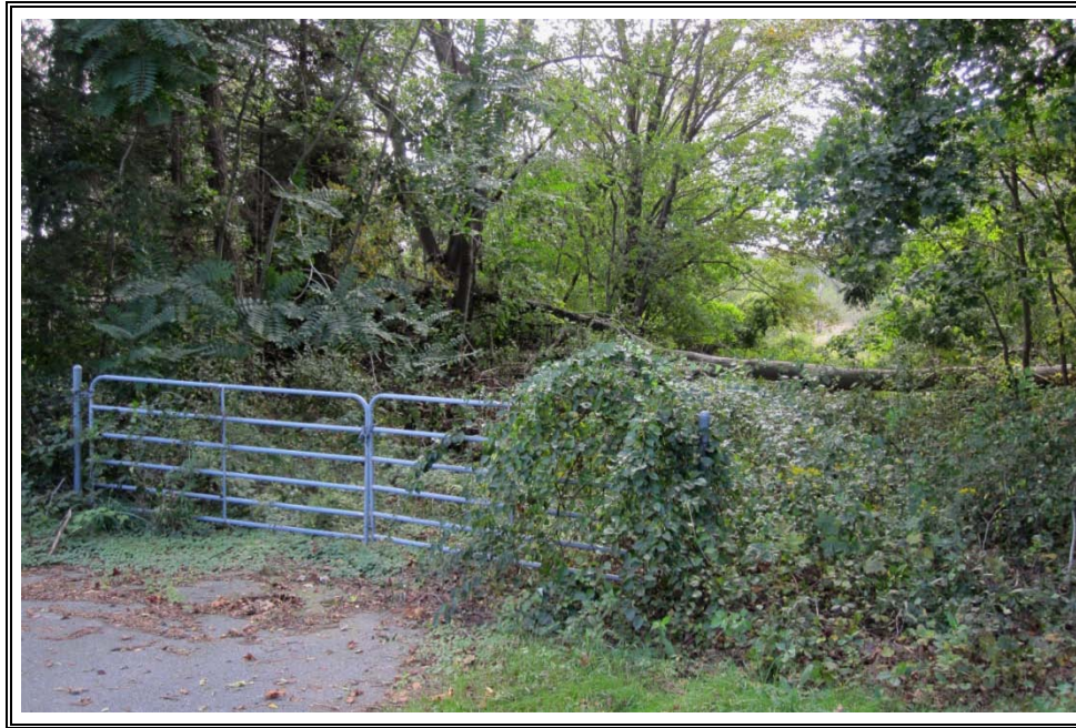
Southeast view of entrance gate at subject's easternmost frontage on Bridge Road
