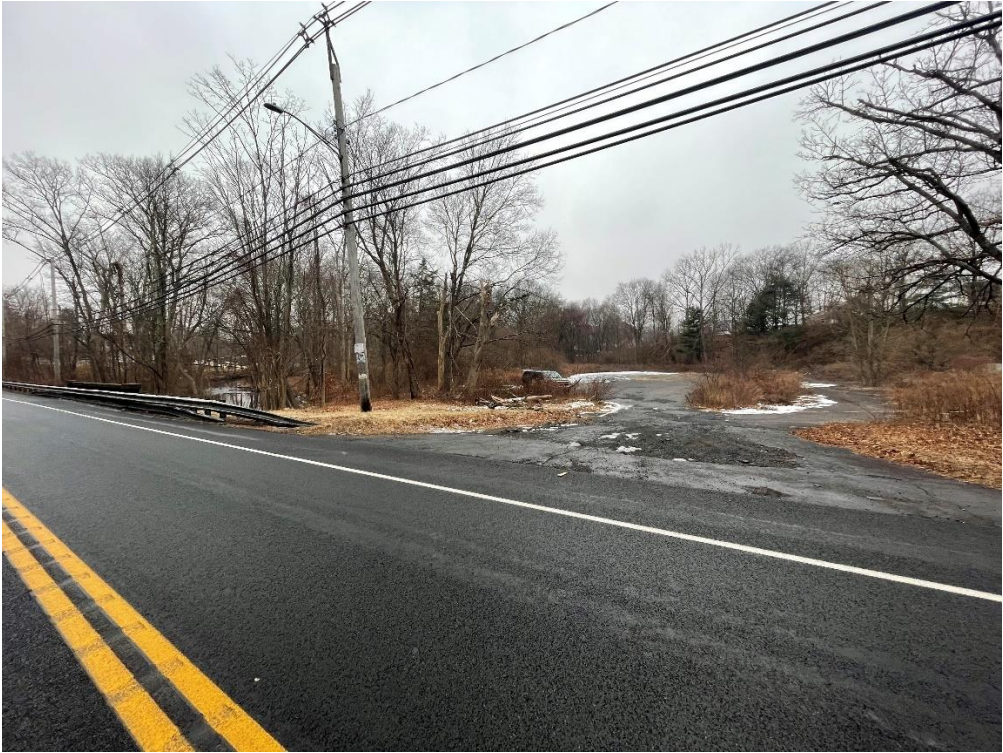
Views from Route 22 looking southwesterly towards driveway into 730 Forest Road, Northford, across DEEP property.
