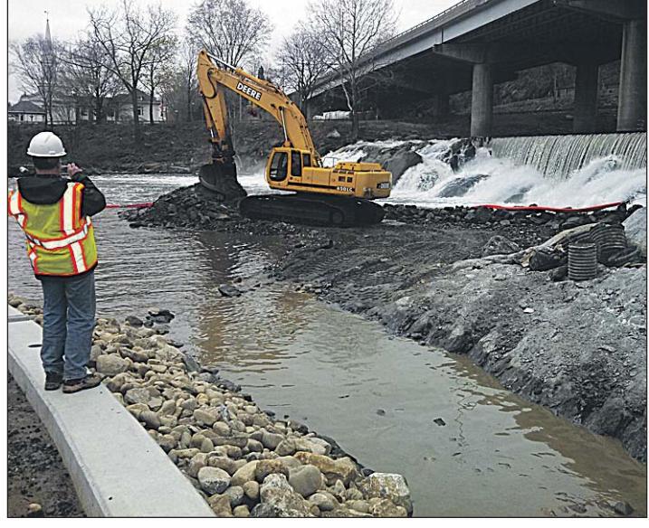
Construction on a fish passage at Tingle Dam in Seymour.
