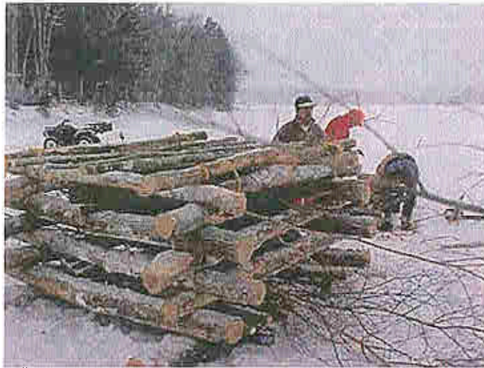
Figure 5. A Wisconsin Style log crib that was constructed on the ice in Wisconsin. http://www.nden.k12.wi.us/grants/photocrib.htm
