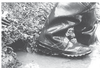
Drive stake in all the way
