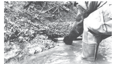
Dig pocket at water line
