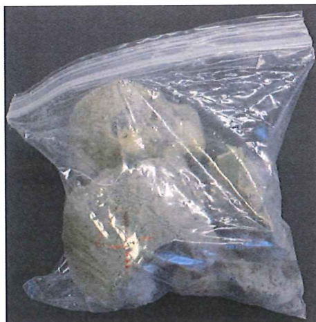
Fig. 4.4 Completely disintegrated core sample of concrete foundation wall– house 1
